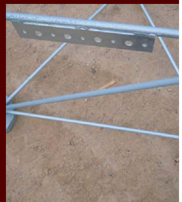
Integral transmission line supports
